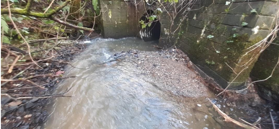
Photograph 11. Sheepwalk Stream Culvert (FW1) (Refer to Appendix 12.4 Sheet 8)
